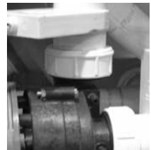
Slice Valve and Pump Union
