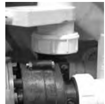
Slice Valve and Pump Union
