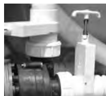
Slice Valve and Pump Union
